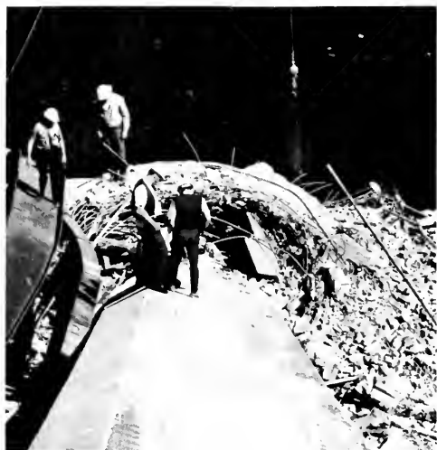
Photo 19. Collapsed column at overcrossing at the Golden State Freeway and State Highway 14 interchange [7].
